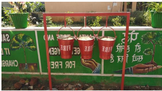
(a) Fire extinguisher
