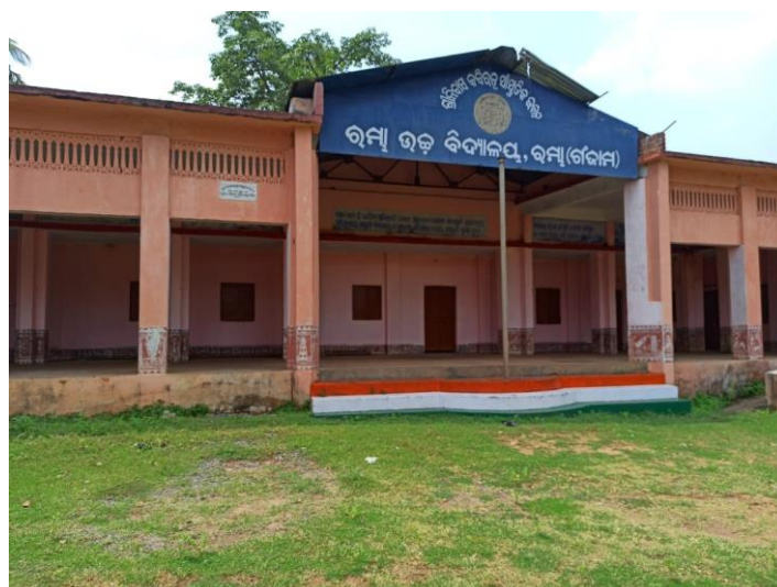
Figure 35: School building, Ward No. 9, Rambha NAC, Ganjam
