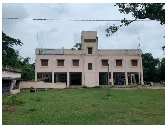
(a) Multi-Purpose Cyclone Shelter, Bolang
