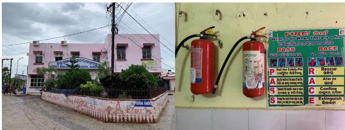
Figure 11: District Headquarter Hospital, Kendrapara and Fire Safety Measures in the Hospital
