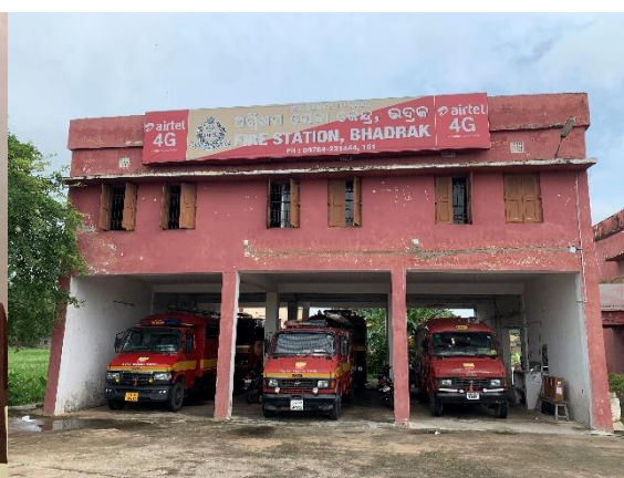
(b) Fire Station, Bhadrak
